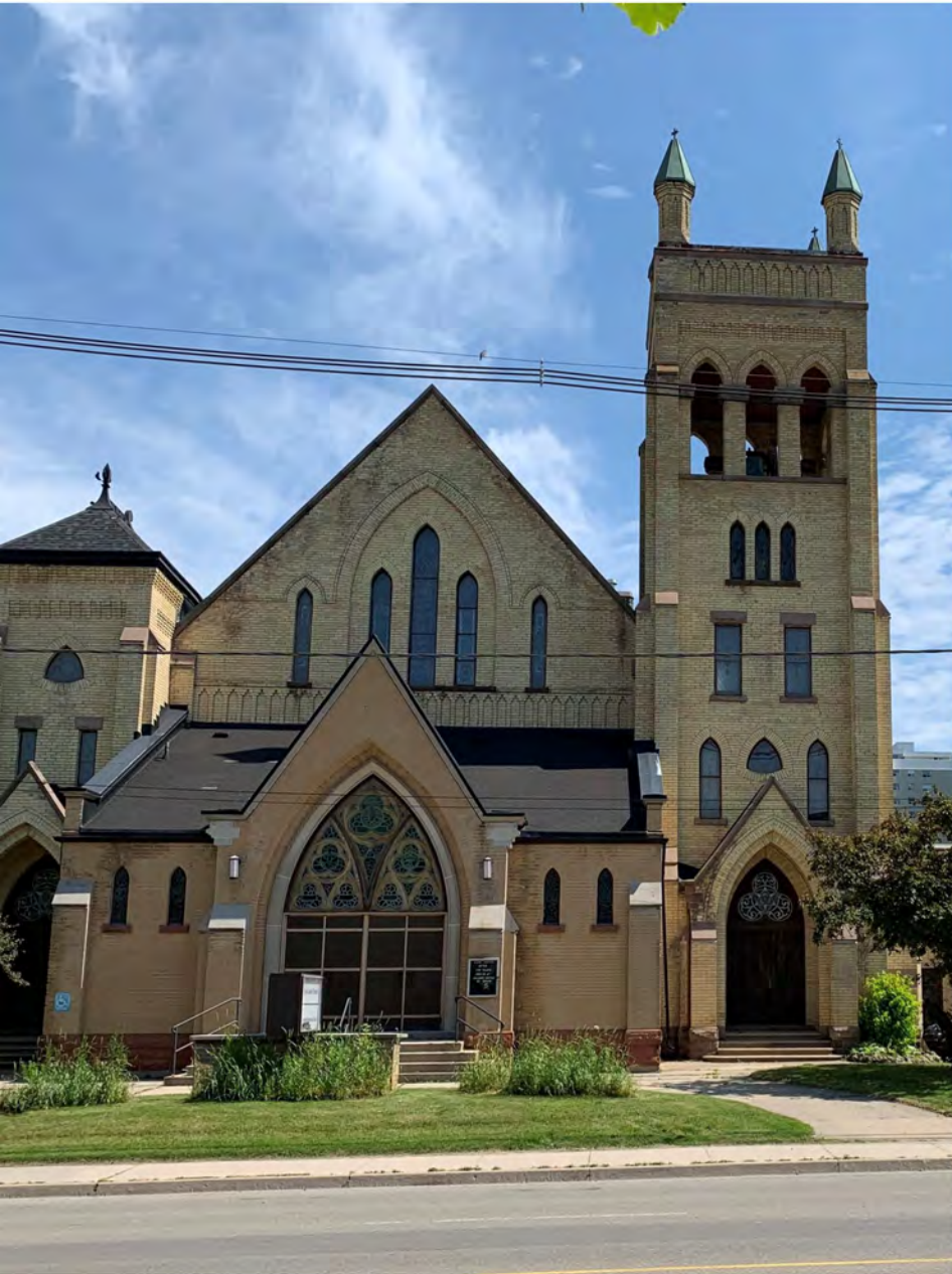
32 WEBER STREET WEST (GROUP B)
