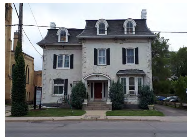
28 WEBER STREET WEST (GROUP B)
