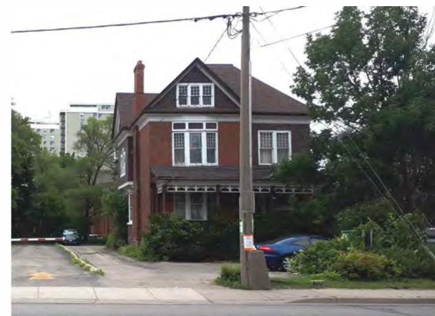
18 WEBER STREET WEST (GROUP B)
