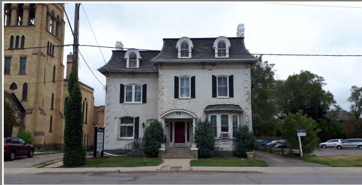
28 WEBER STREET WEST LOCATED IMMEDIATELY WEST OF THE SUBJECT LANDS IS USED AS AN OFFICE.
