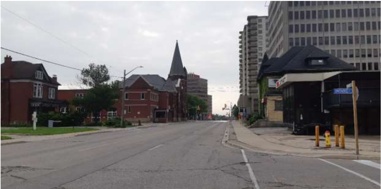
Figure 18 – View of higher density development and contemporary buildings located south-east of the subject property near the intersection of Queen Street and Weber Street (Source: MHBC, 2019)
